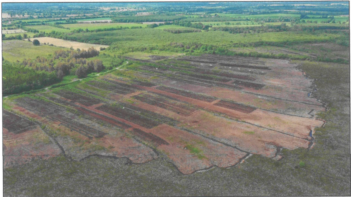
Figure 2: DRAINAGE AND PEAT REMOVAL FROM SOUTHERN SECTION OF BOG
